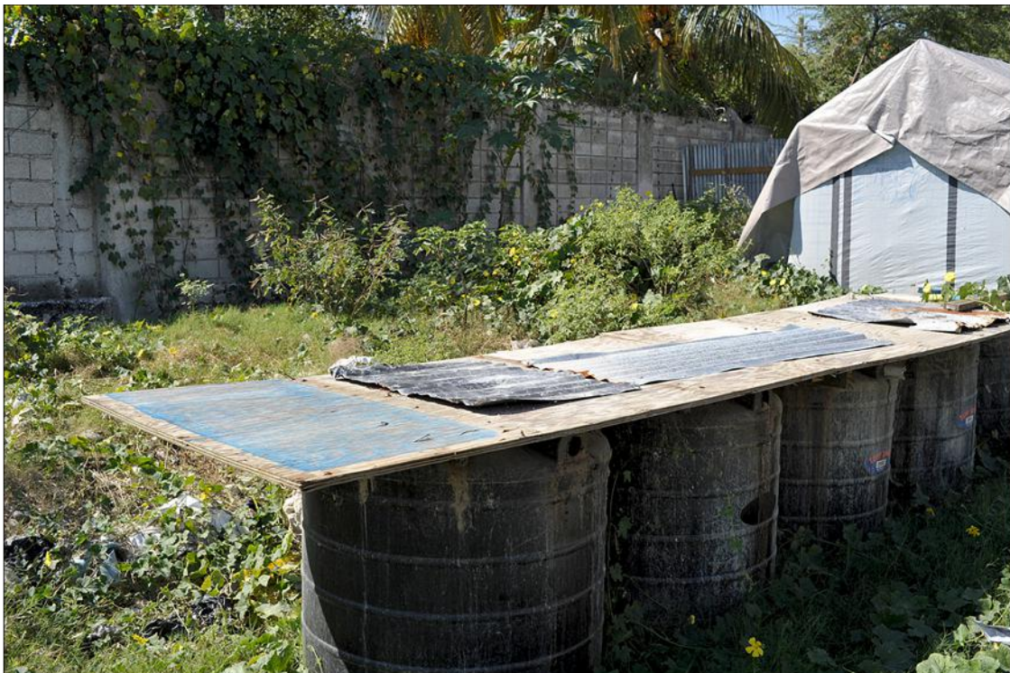
Below: Covered, black latrine tubs holding waste at Camp Blue in Port-au-Prince.
